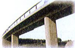
a concrete bridge
